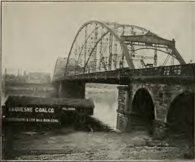
SIXTH STREET BRIDGE
